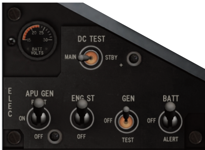
Fig. 16 Electrical Power Supply Panel
